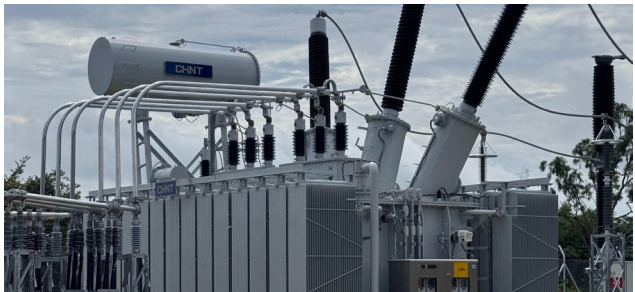
Colombia | 180 MVA 220 kV Natural Ester Transformer
