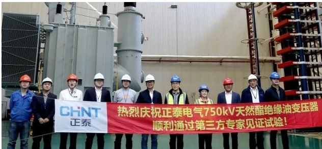
China | 750kV Natural Ester Transformer Type Tests Successfully Witnessed by Third Party Experts
